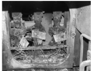
Fig.16 Cofret relee maximale de curent poz.54.1-3
